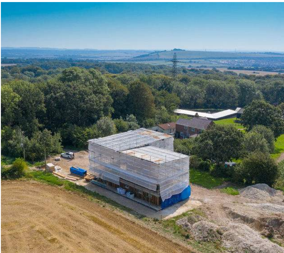
Full scaffold with tin hat and monarflex sheathing
